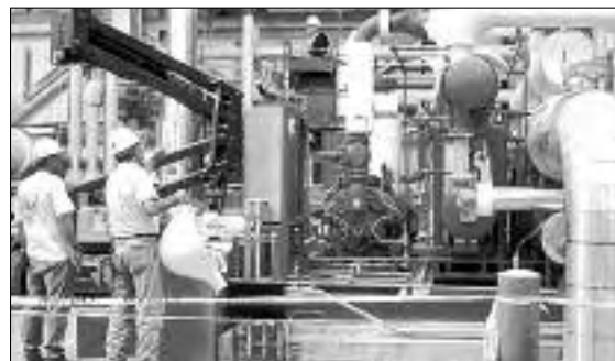
LOCAL 12 PLUMBERS on the job.
